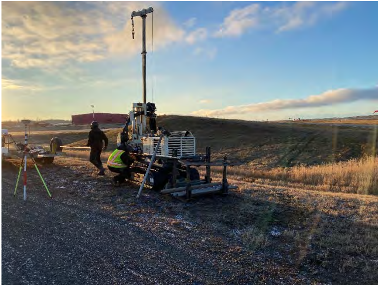
Typical soil boring installation
