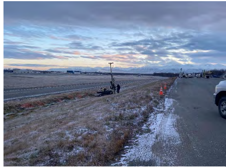
Typical drilling setup
