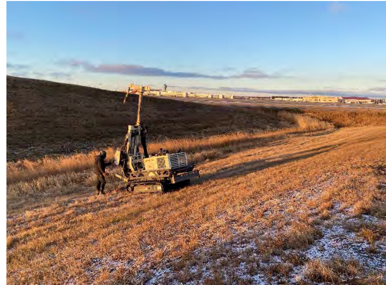
Drilling along Side Slope
