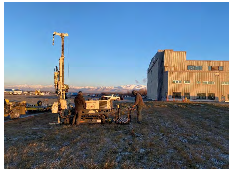
Typical drilling - looking east
