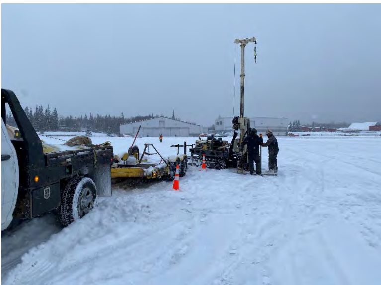
Typical drilling setup along Taxiway
