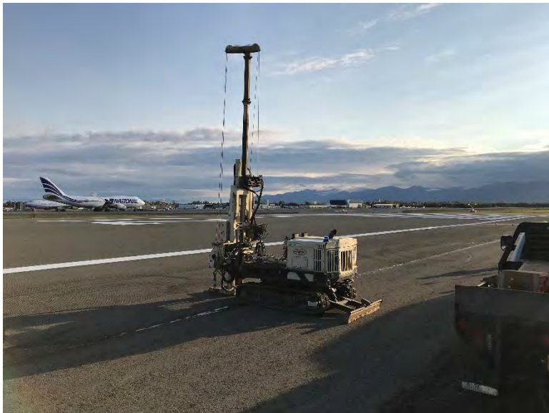
Typical drilling setup along taxiway
