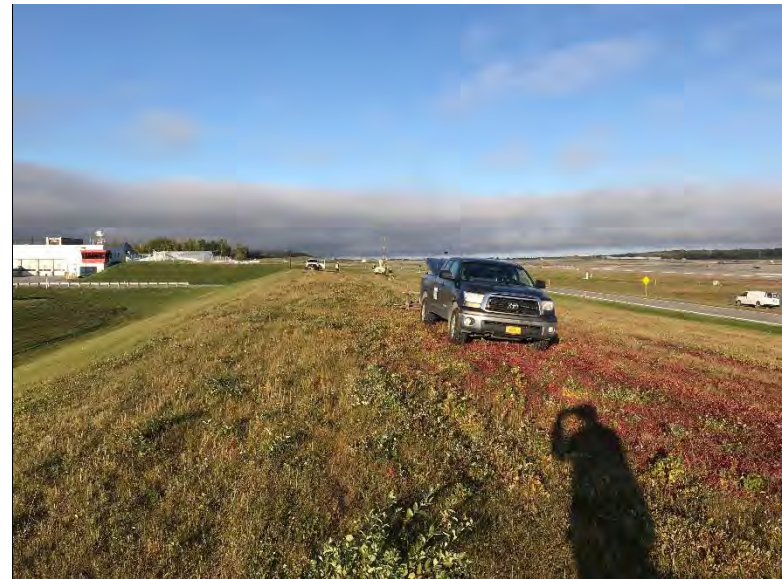
Drilling along the proposed Tug Road – looking west
