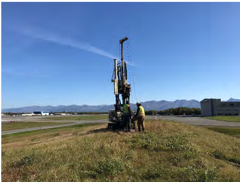
Drill rig setup along proposed Tug Road
